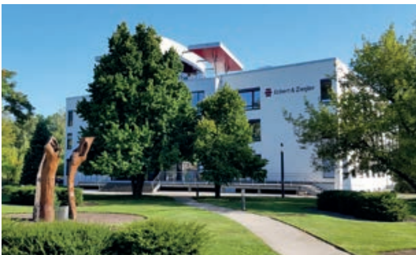
Energy-efficient corporate headquarters in Berlin-Buch
